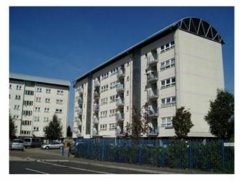
By the 1980's it was obvious that the estate was suffering from design and construction problems causing water penetration and massive condensation problems to many flats. Although the flats were of generous standard, they were poorly insulated and the technical shortcomings in design and construction had led to severe condensation problems and to extensive water penetration through leaking roofs and cracking walls
