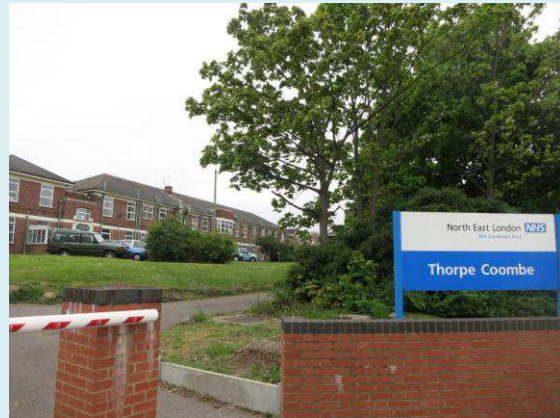
Above: Some of the hospital extension.
